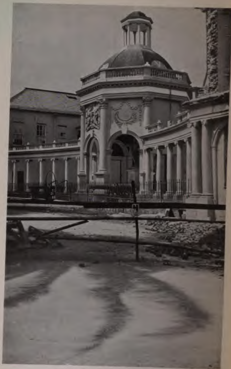
RODNEY'S MONUMENT, SPANISH TOWN. The damage done by the earthquake will be noticed.
